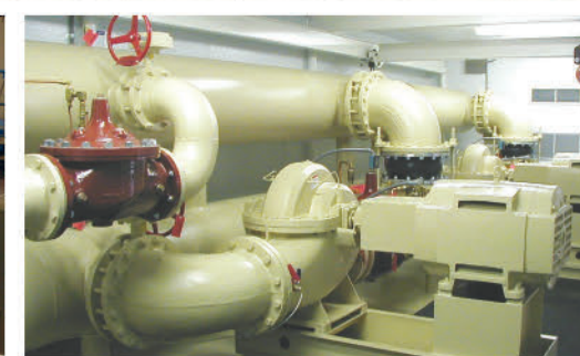
HORIZONTAL SPLIT CASE WITH BRIDGE CRANE
