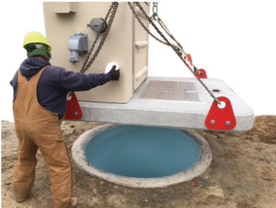
One-piece valve & control station that is fully assembled at factory. Fits wetwells 5-12 ft diameter.
