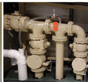
Manual air release valve
