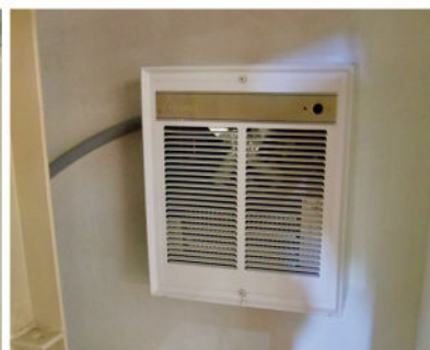
Thermostatically controlled wall heater and exhaust fan.
