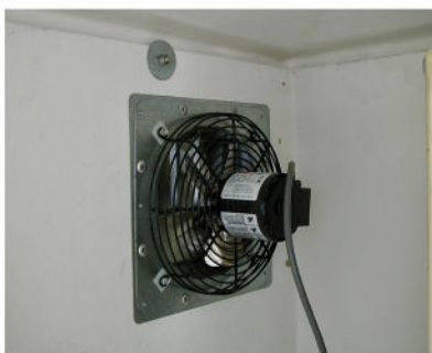
Thermostatically controlled wall heater and exhaust fan.
